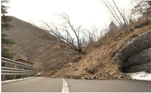
Trees prevent soil erosion.
